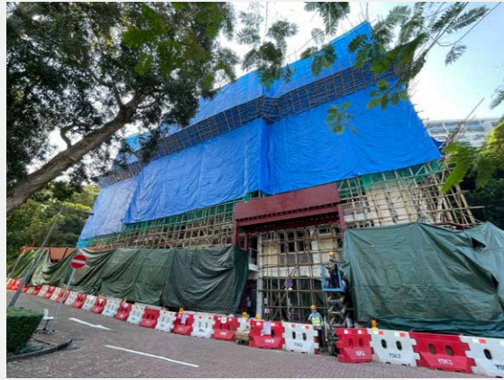
11.2023 外圍搭建竹棚並蓋上帆布 Bamboo scaffolds and canvas set up
