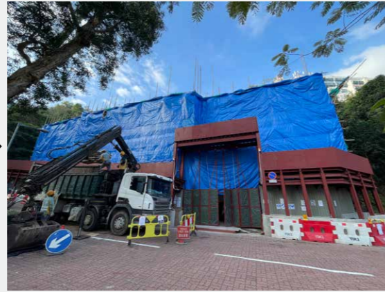
12.2023 開始拆卸 Demolition started
